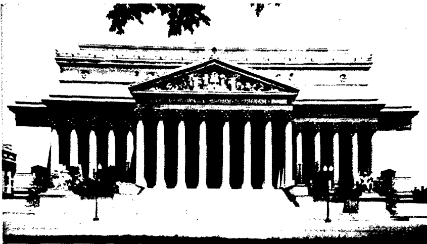
National Archives Building, Washington, D. C.
