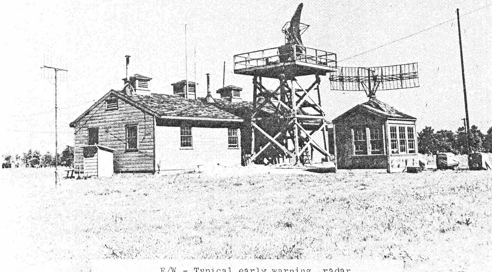
E/W - Typical early warning radar station showing AN/TPS-10A height finder on left and AN/TPS-1B search radar on right.
