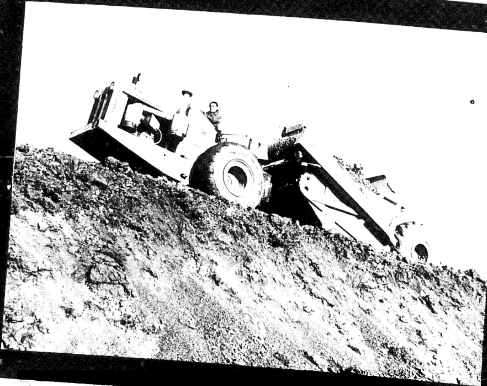
Large earth movers toil on Upper Heyford's airfield clearing tons of dirty and rock away to make way for workmen during the month of November 1957. The earth movers are a part of the force being used during the Payment Strengthening Project.
