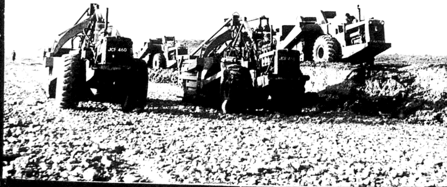
Giant earth movers work on Upper Heyford's airfield during the month of November 1957, moving tons of earth and leveling various areas. This is part of the SECRET DECLASSIFIED IAW EO 13526 program.
