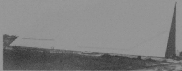
AN/FPS-85 phased array radar system at Eglin AFB, Fla.
