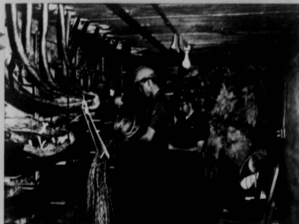
SSgt. R. Rather (241st) and Sgt. C. Fiore (213th) splice telephone cables at Kadena AB.
