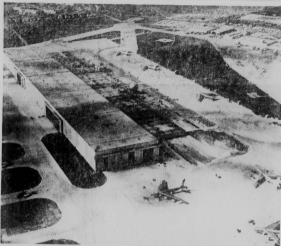
CONTINUED GROWTH — Giant maintenance hangar at Kelly Air Force Base houses the same mission—as the tents that were strung up in a makeshift patch 50 years ago.
