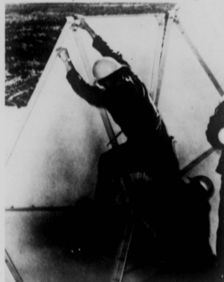
PIECE BY PIECE . . . Personnel of the 2861st GEEIA Squadron match holes in adjacent panel prior to bolting the panel in place.
