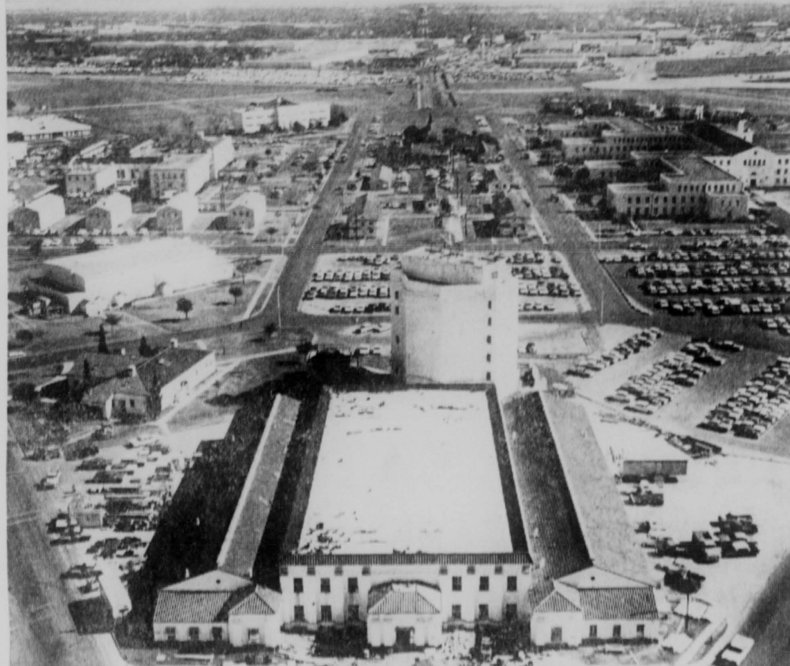
THE STRUCTURE (foreground) is the new Kelly Comptroller Bldg. in the completion stages. The two-story structure will provide 60,000 square feet of modern office space for the 550 comptroller personnel of SAAMA at Kelly AFB.
