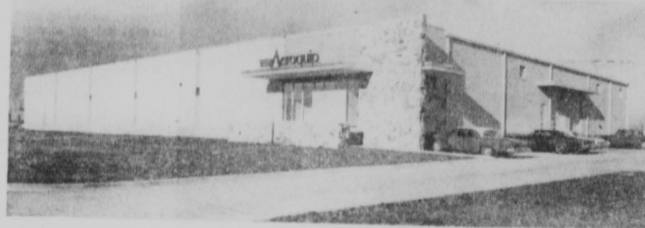
Aeroquip's Dallas plant is located at 1261 Profit.
