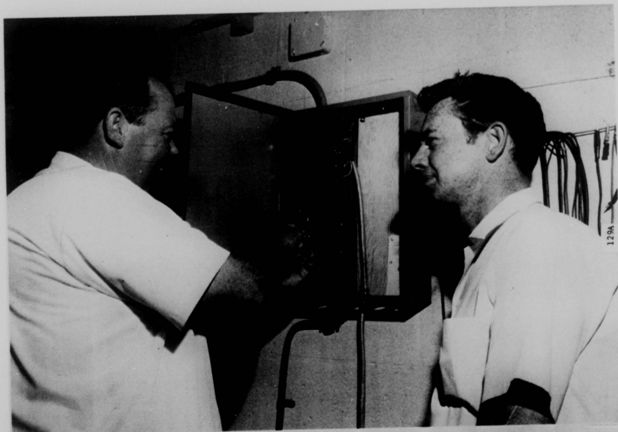
2166-69 AFFTC UNCL SURGE PROTECTION INSTALLATION TERMINAL BOX
