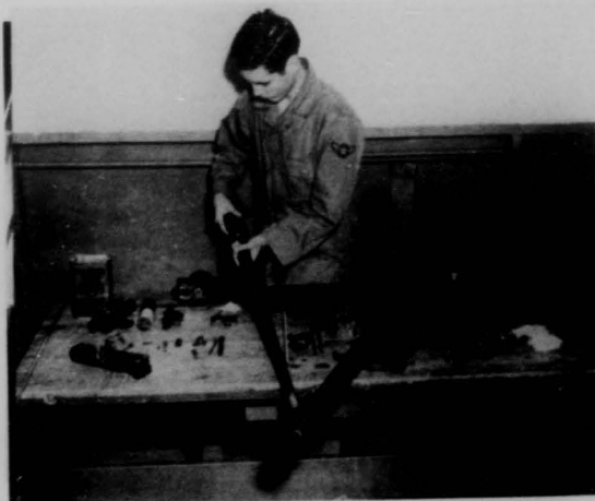
Disassembling the .50 caliber Browning in the classroom. Student gunners spent many hours in this vital training, designed to impart knowledge and skills that came in handy many times in crucial combat situations. Smithsonian Institution
