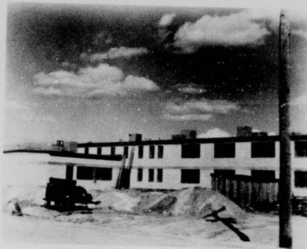
A view of the new Operational Readiness building which was under construction during the period.
