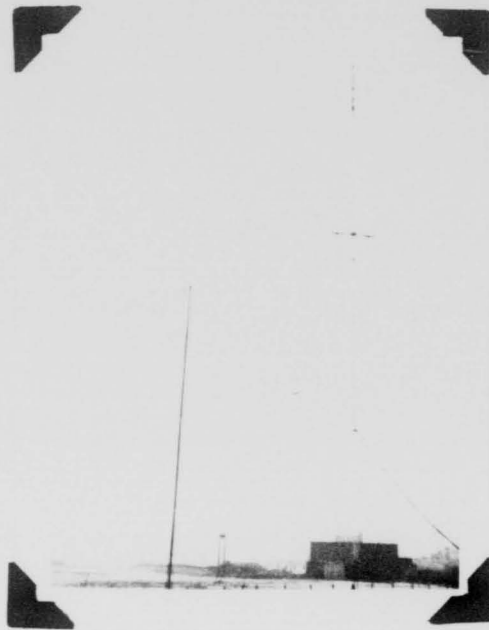
Photo 5. AN/TRC-27 antenna Mast. Note AN/TRC-11 antennas at Sixty Foot Level.
