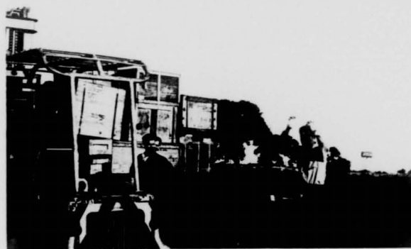
Photo 11. Moving equipment out of coal bin.
