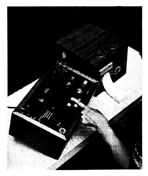
Figure 5. ESP Teaching Machine used in this experiment. An incorrect choice of target is indicated. Two of the five "encouragement lights" at the top of the machine are illuminated. The printer to the right of the machine records data on fan-fold paper tape.
