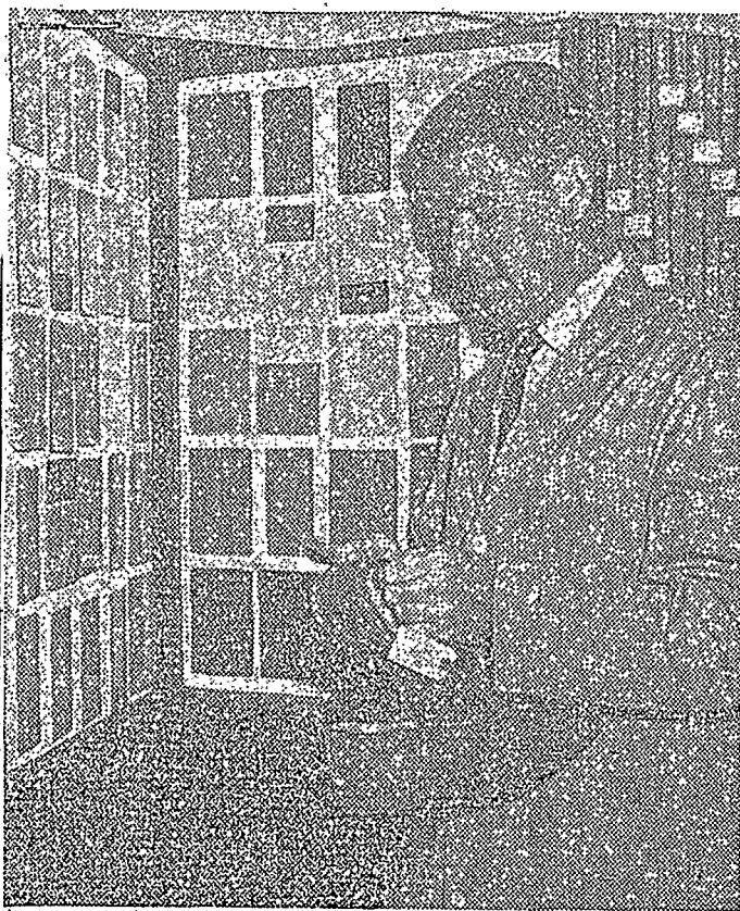
CRIME DETECTOR —The FBI Laboratory has developed scientific crime detection to a fine point. This researcher is checking paint on shoes of a hit-run victim against panels showing paint of every model of American car.—AP Photo.
