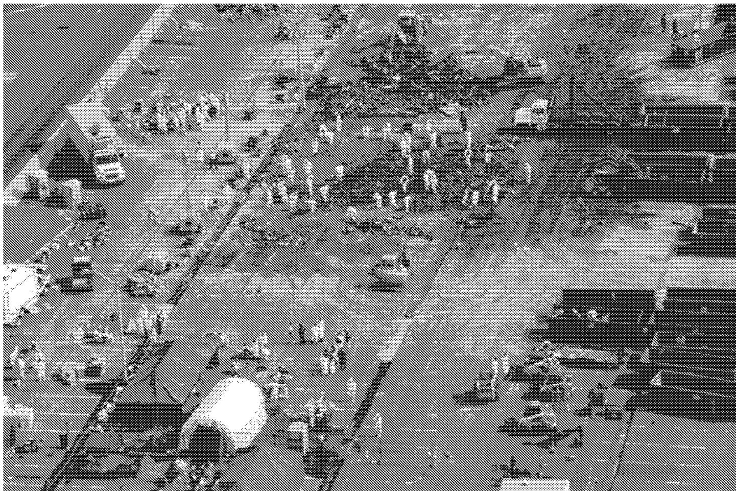
Crews work in the rubble pile in the North Lot of the Pentagon. (Photo courtesy of the Washington Field Office)
